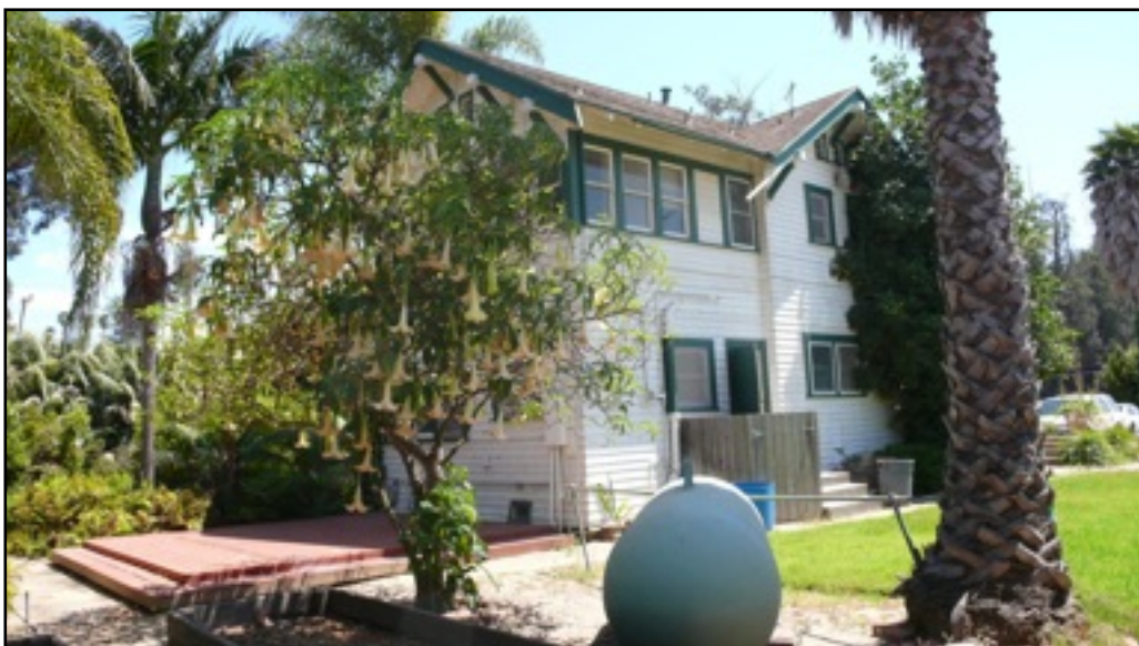
Photo 3. Residence, northern and eastern elevations. [6-28-2011]
