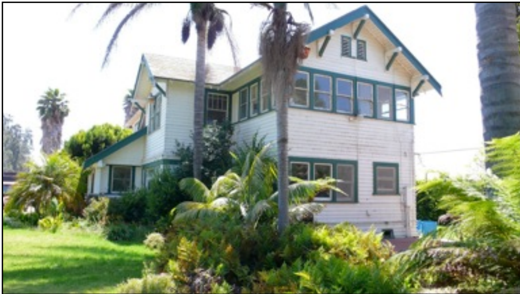
Photo 2. Residence, souther and eastern elevations. [6-28-2011]
