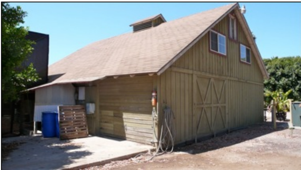
Photo 6. Walnut dehydrator, southern and western elevations. [6-28-2011]
