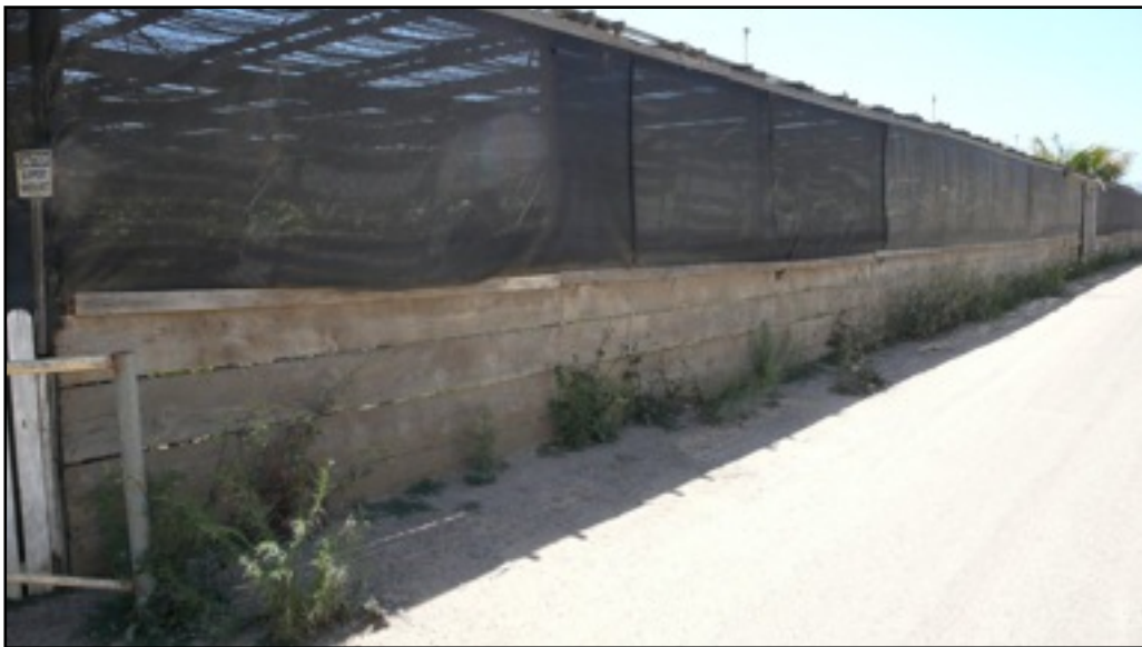
Photo 8. Shade buildings, representative example, viewed from southeast. [6-28-2011]
