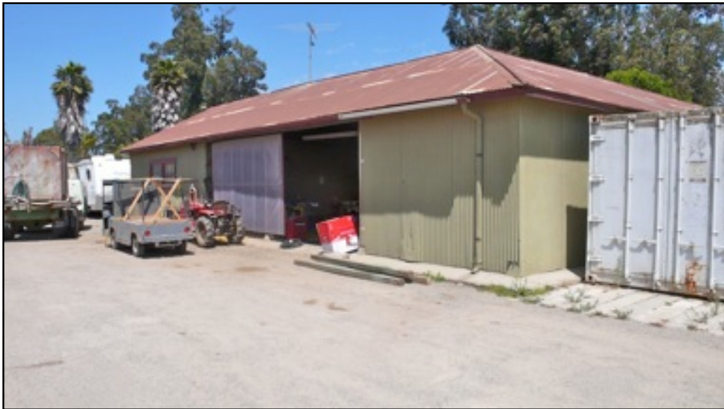
Photo 5. Shop/storage/equipment shed building, northern and western elevations. [6-28-2011]
