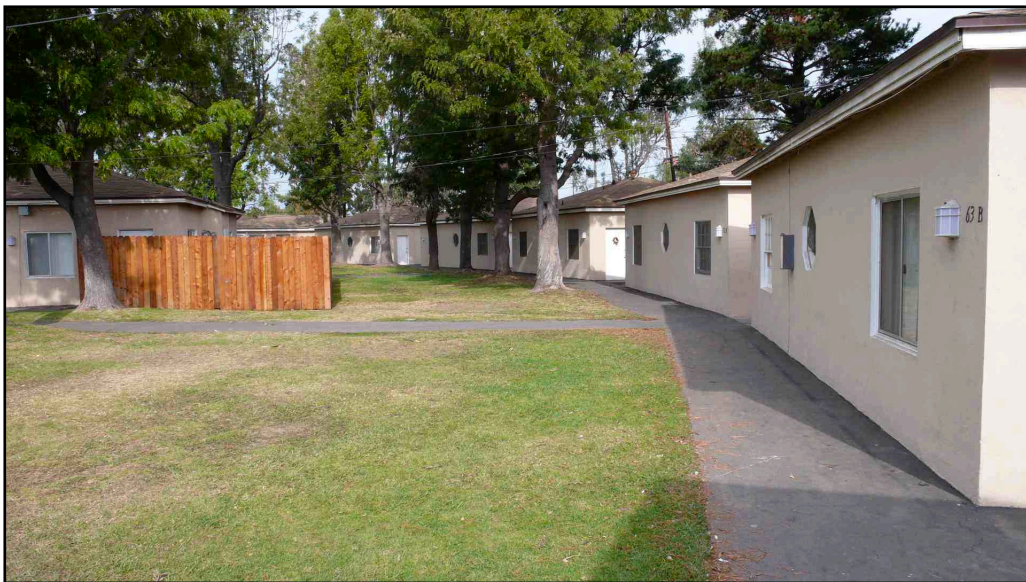
Photo 6. Duplex unit arrangement, typical. [5 December 2007]
