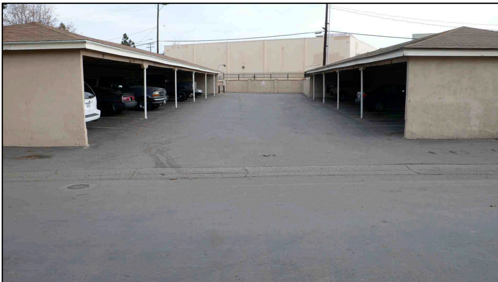
Photo 12. Carport buildings, typical. [5 December 2007]
