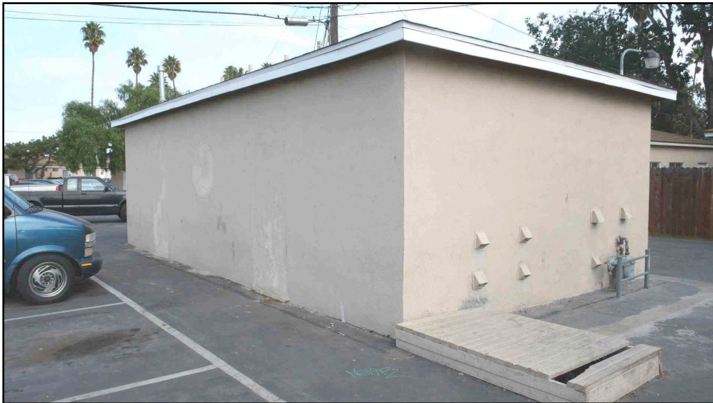
Photo 11. Laundry room building. [5 December 2007]
