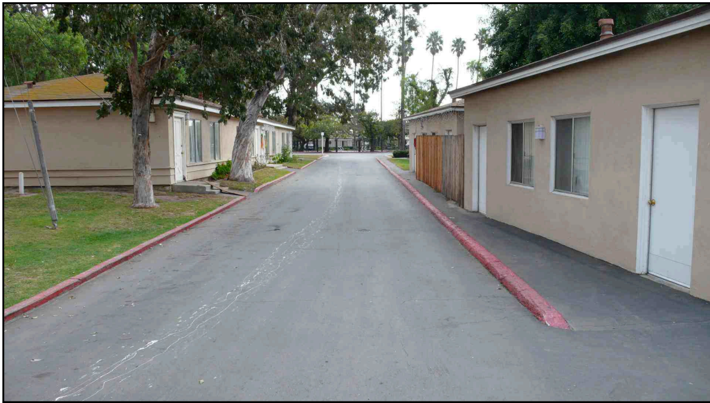
Photo 8. Type 1 apartment building on left, duplex unit on right, driveway viewing southeast. [5 December 2007]
