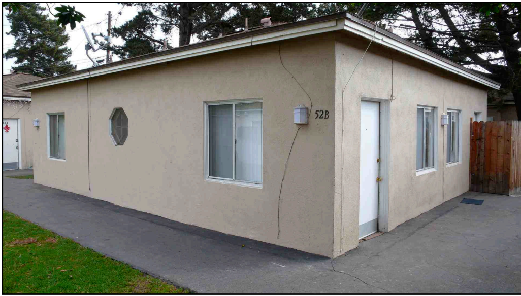
Photo 4. Duplex unit, typical. [5 December 2007]
