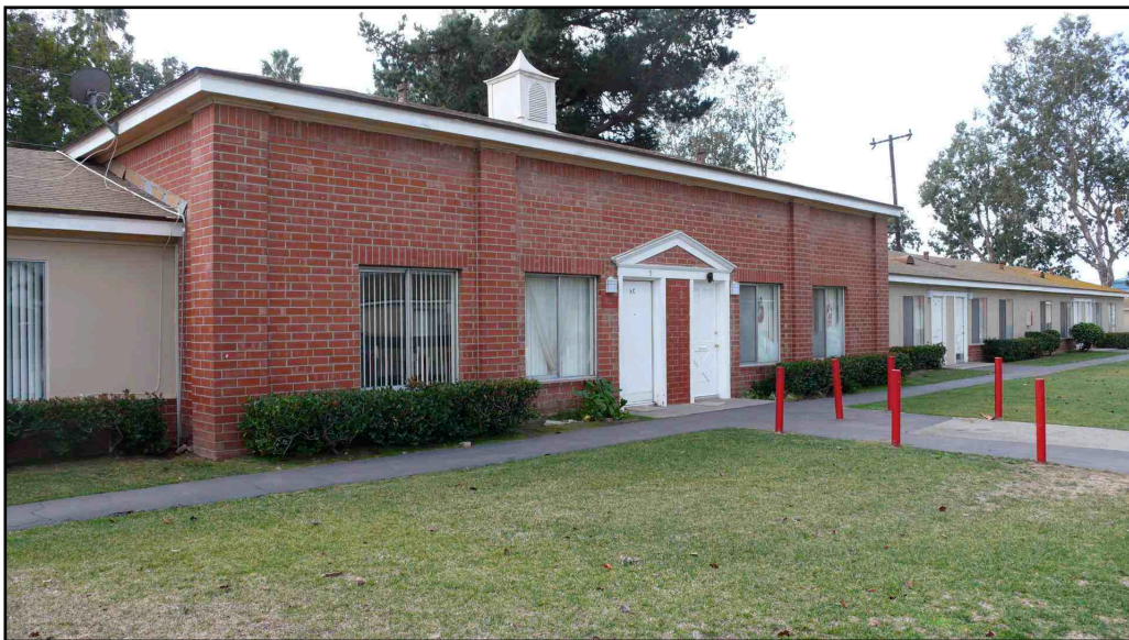
Photo 9. Type 2 apartment building, typical main elevation. [5 December 2007]
