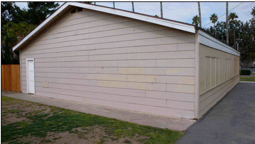
Photo 3. Storage building, southern and eastern elevations. [5 December 2007]
