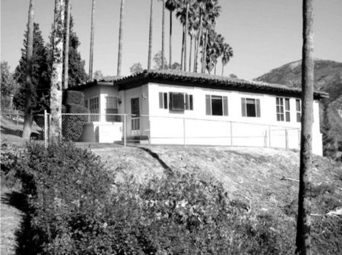
PHOTO 10. Bungalow 9, northern and western elevations (6 Nov 2004).
