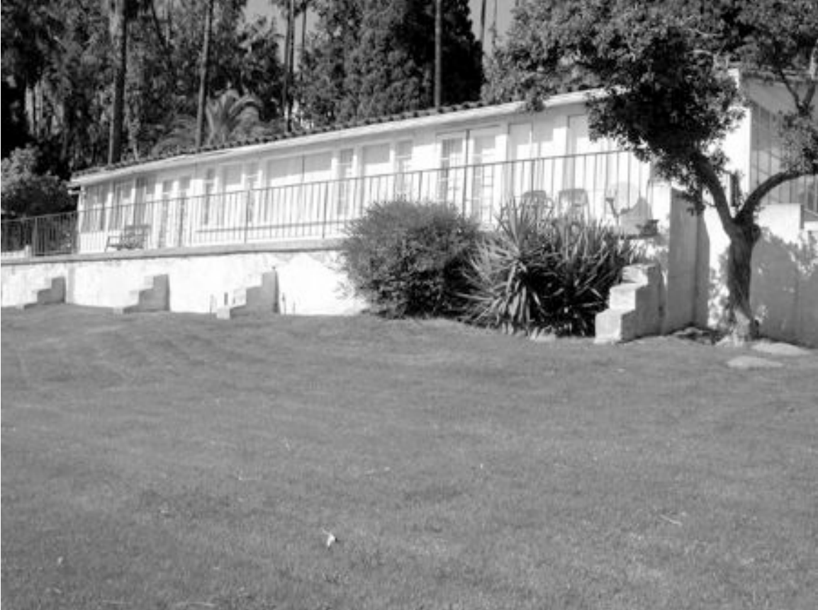
PHOTO 8. Bungalow 7, southern elevation (6 Nov 2004).
