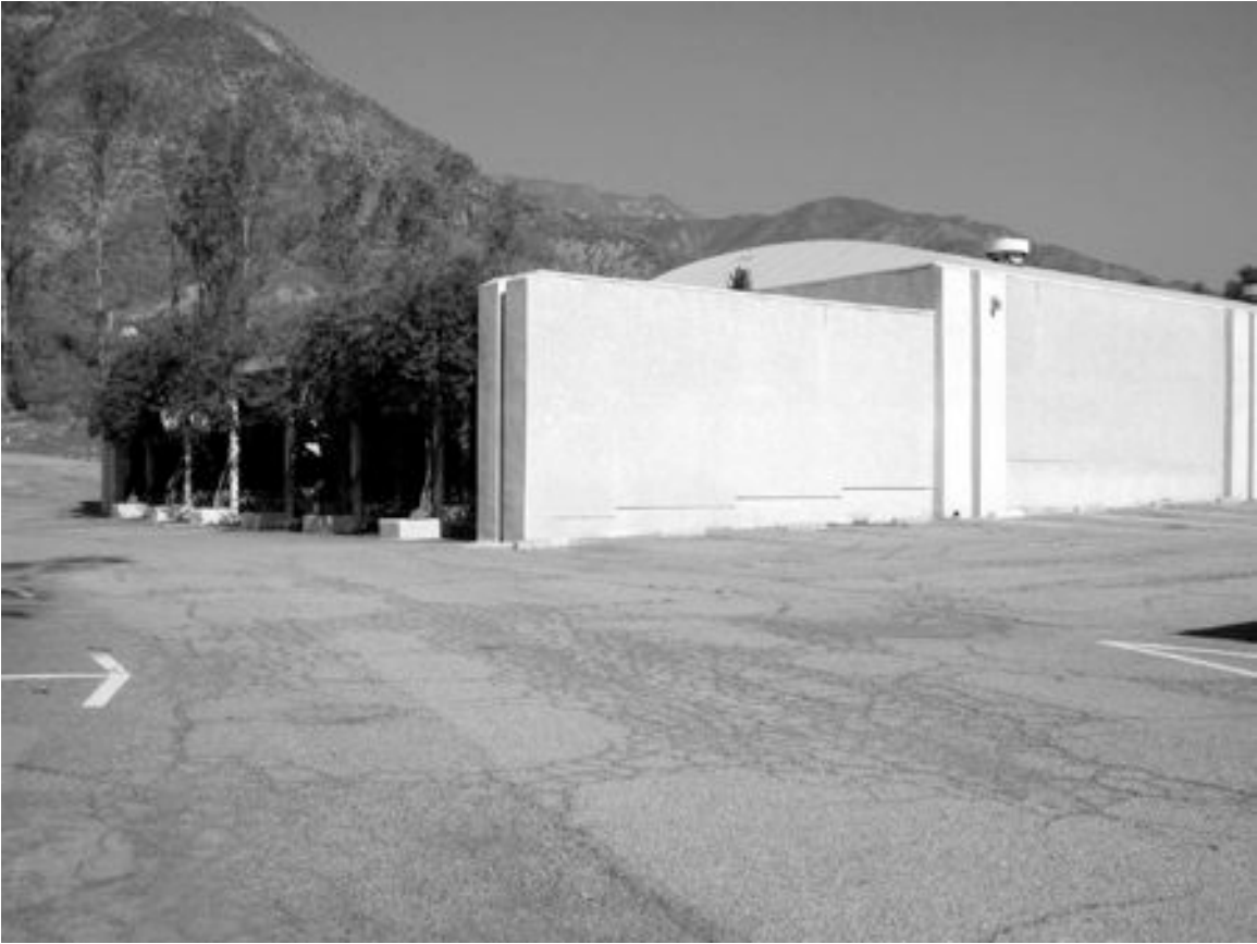
PHOTO 13. Garage/Hill Auditorium, southern and western elevations (6 Nov 2004).
