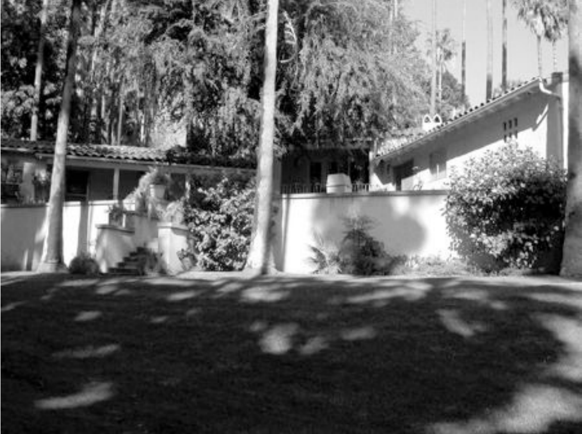
PHOTO 6. Bungalow 1, southern elevation (6 Nov 2004).
