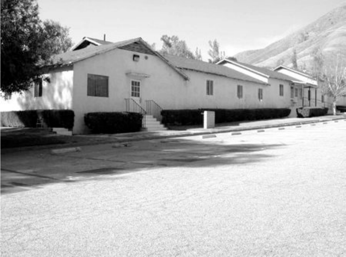
PHOTO 14. Hacienda, eastern elevation (6 Nov 2004).
