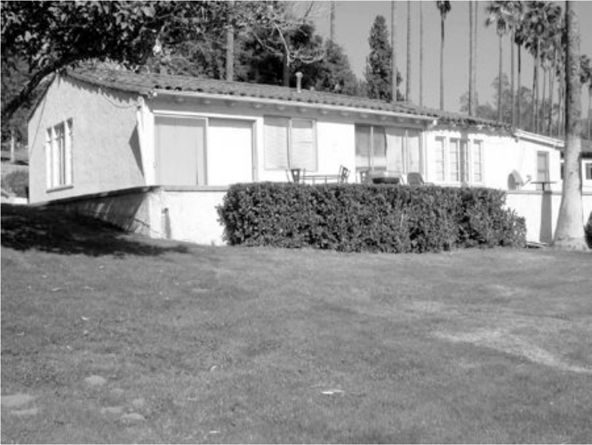
PHOTO 9. Bungalow 8, southern and western elevations (6 Nov 2004).
