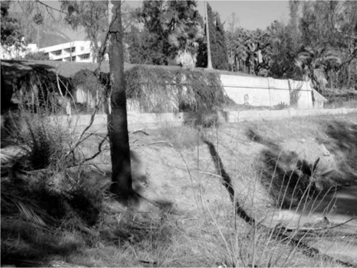
PHOTO 19. Terrace, viewed from southwest. Northwestern corner of tennis courts visible in right foreground (6 Nov 2004).
