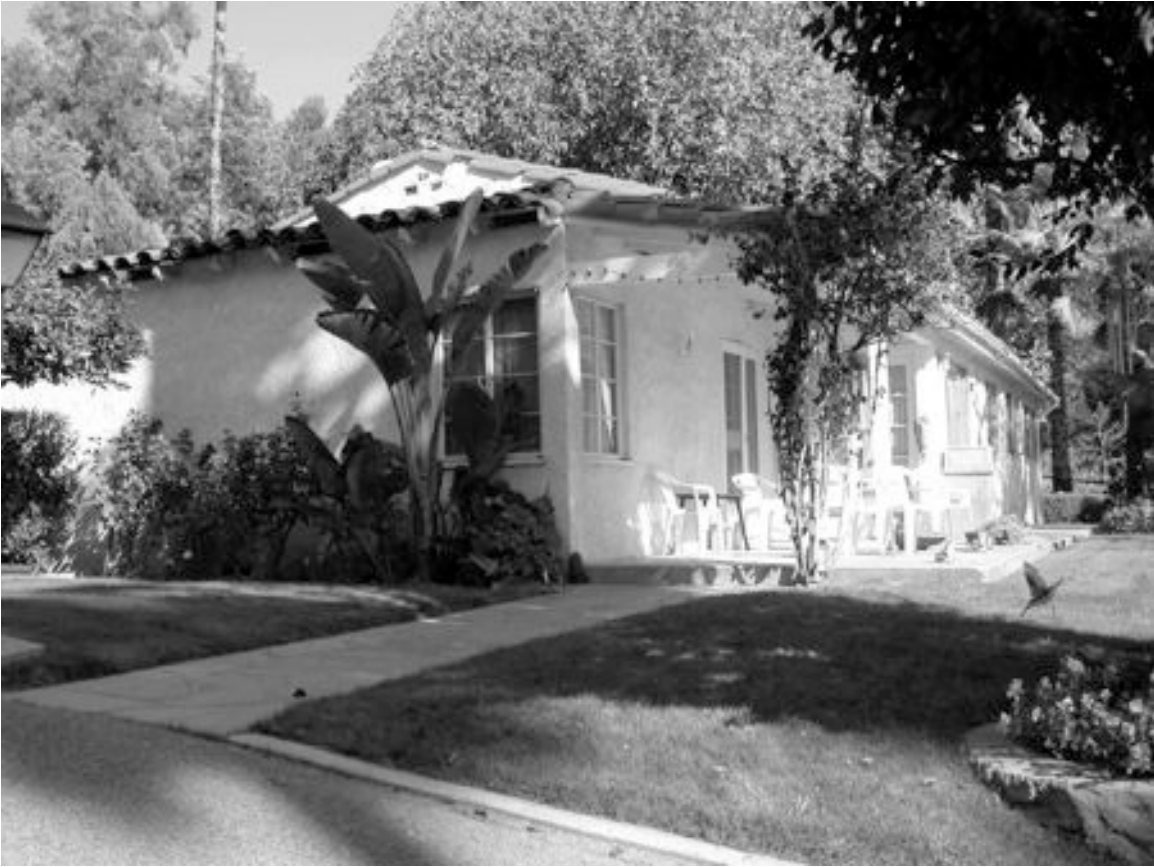
PHOTO 7. Bungalow 4, western and southern elevations. (6 Nov 2004).
